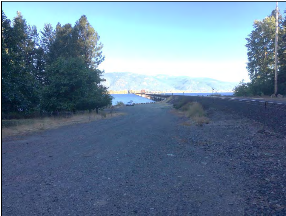
Figure 18. View of Conditions South of 10BR38, Showing Modifications Since 2008; View to Northeast
