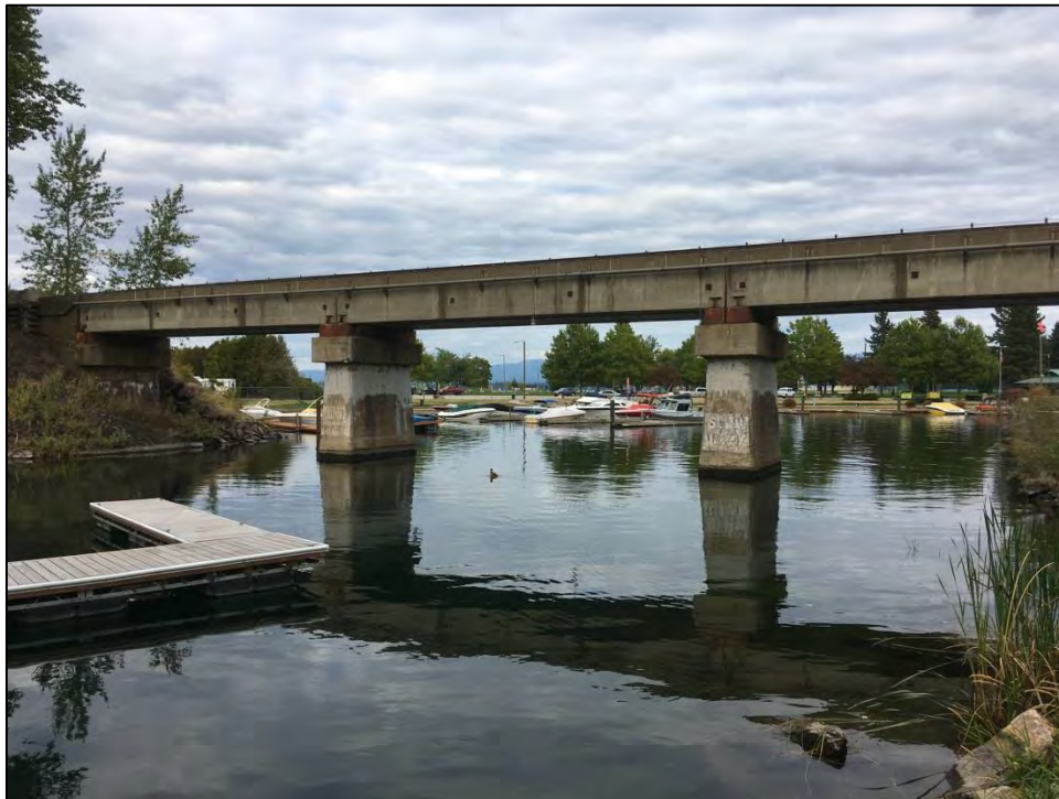
Figure 32. BNSF Bridge 3.1, West Elevation
