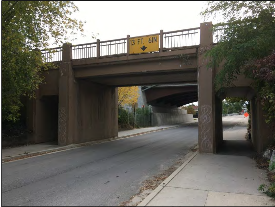
Figure 28. BNSF Bridge 3.0 West Elevation
