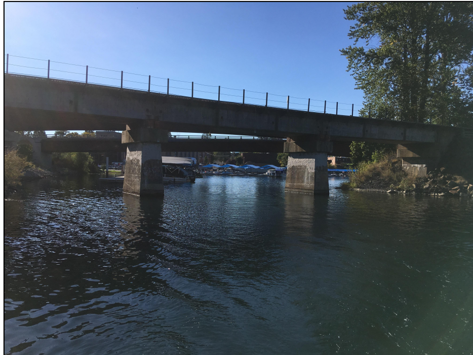
Bridge 3.1, East Elevation
